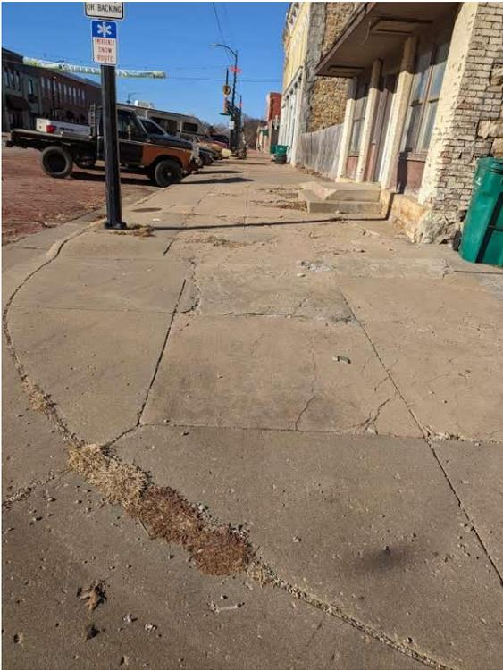
North Sidewalk of Broadway Street (looking west towards Sycamore Street) – Current condition of existing radial ramp and pavement
