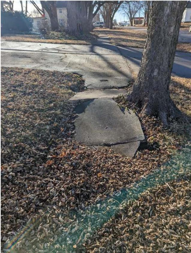
Sycamore Street (looking south towards 3<sup>rd</sup> Street) - Broken sidewalk caused by a tree
